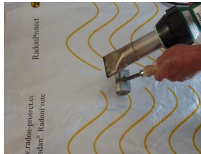
RadonProtect Foil, welding by hot air gun
