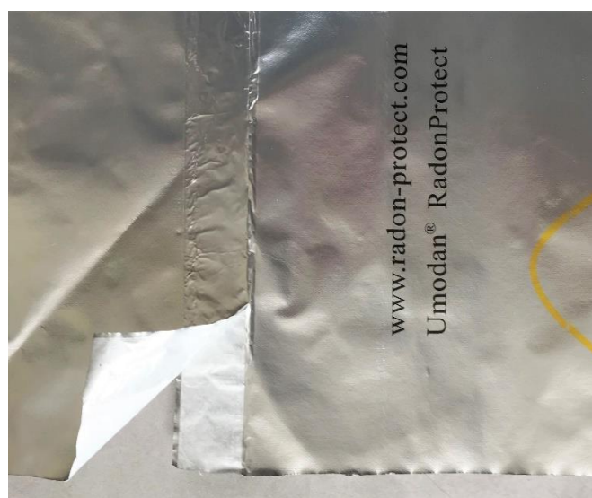
The film strips are glued together using the self-adhesive strips integrated on both sides
